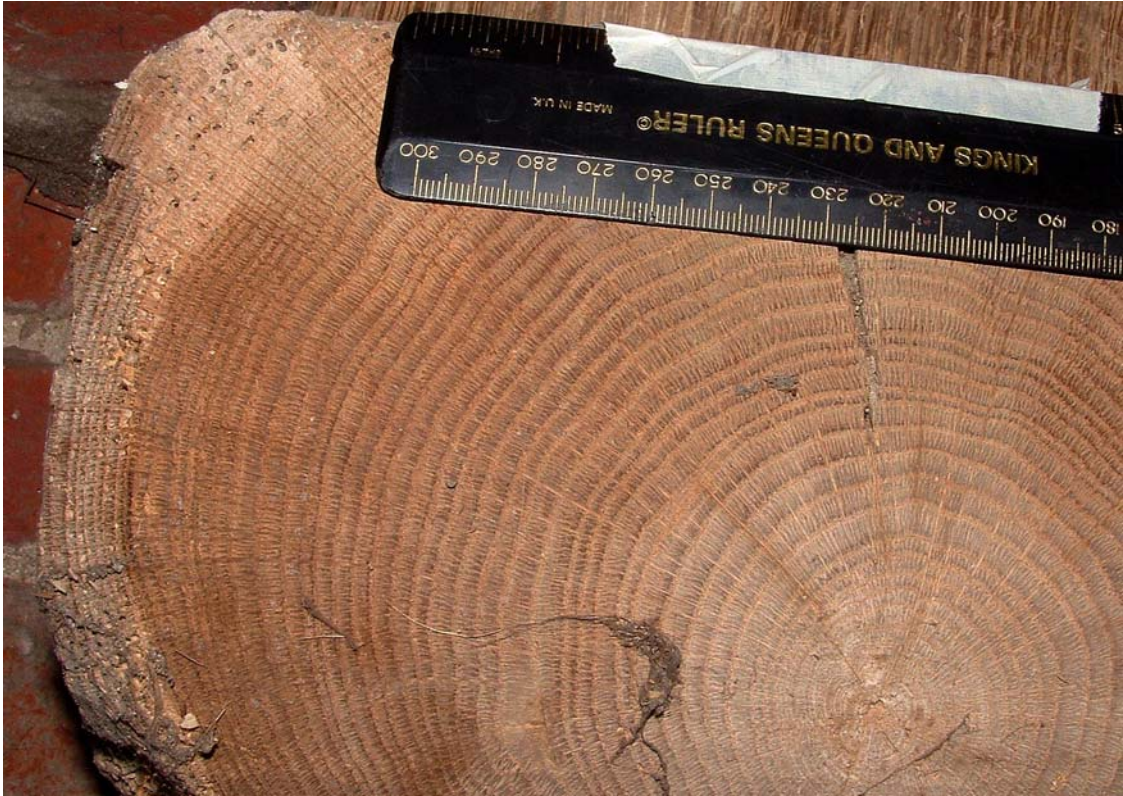
Figure 3: Photograph of HOW06 , the corbel to truss 7 on the south side
